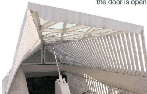
Walls become hyperbolic paraboloids when the door is open
